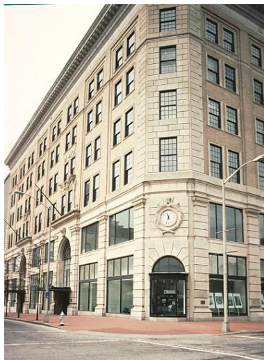
Rich's Department Store (Sam Nunn Federal Office Center)
